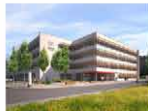
Newry Community Treatment & Care Centre
